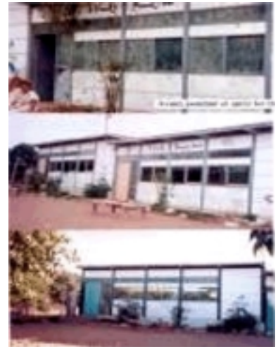
Ecole de Rekkada
